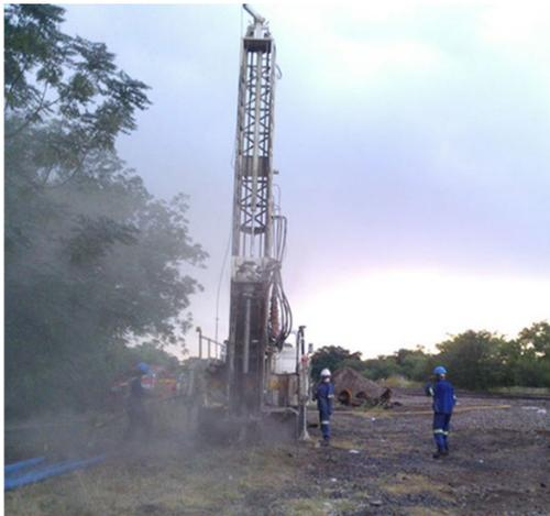
Figure 4 Air rotary drilling Note, in many cases a water well drilling rig is used (note dust) Aqua earth website
