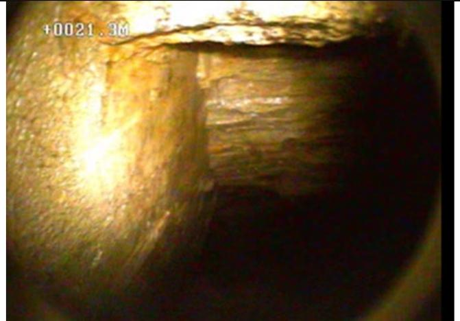
Figure 13 Side view of roof joint intersection in unflooded workings
