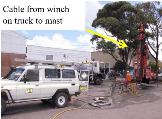
Figure 7 Unstable borehole conditions - Lower device through drill rods with rig on the borehole
