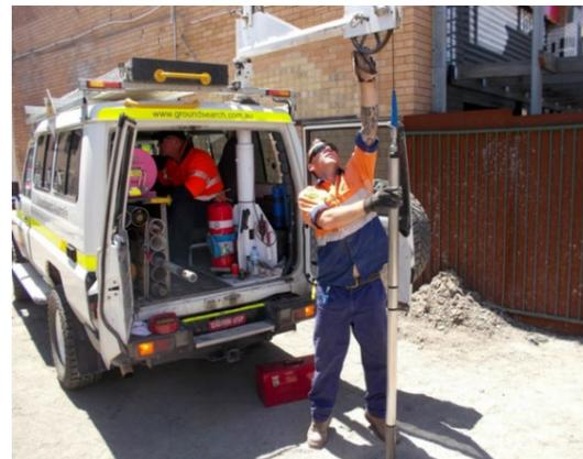
Figure 8 Stable borehole conditions - Lower device through casing in soil zone after drilling
